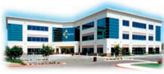
Our new facility in San Diego, CA.
