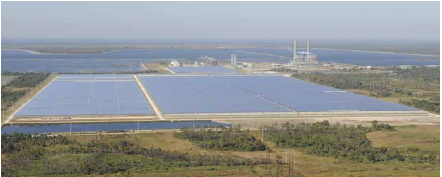
75-MW Martin Solar Plant near Indiantown, Florida
