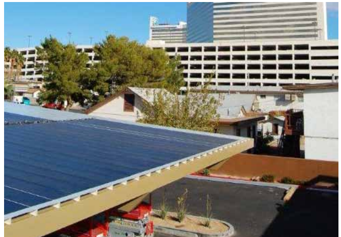
Above: Photovoltaic carport awning in Las Vegas, Nevada
